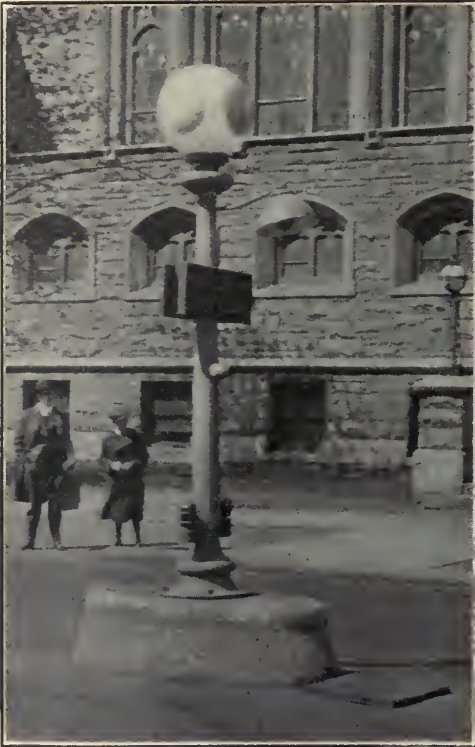
POST WITH TWIN BASE LIGHTS AND GOOSE-NECK TO SHOW OFFICER
